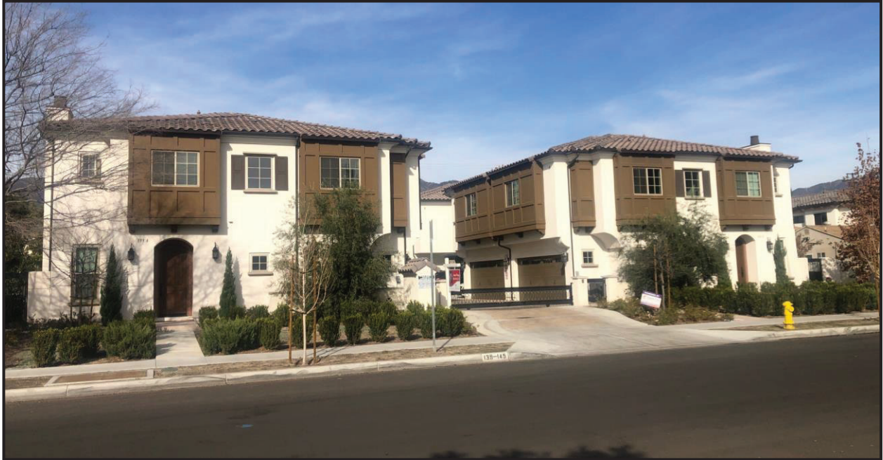
141 – 145 Alice Street – West neighbor next door
